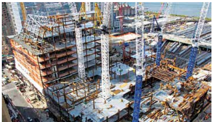
Tower crane, New York, Hudson Yard
