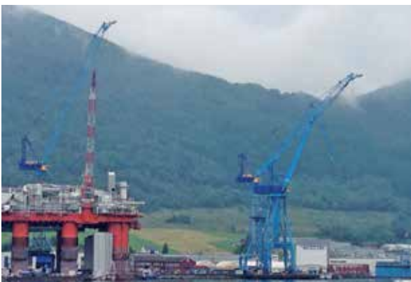
Wharf crane, Norway, Westcon Shipyard
