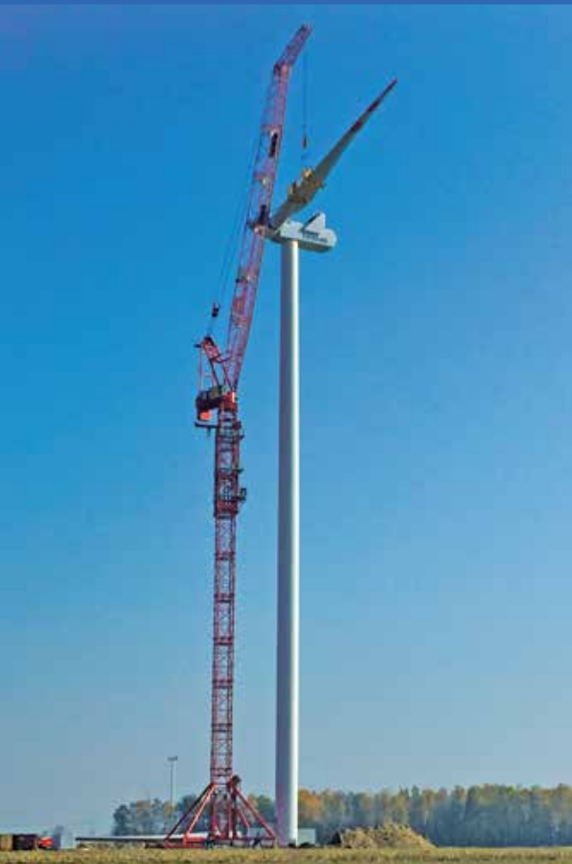
Tower crane, Poland, windmill installation
