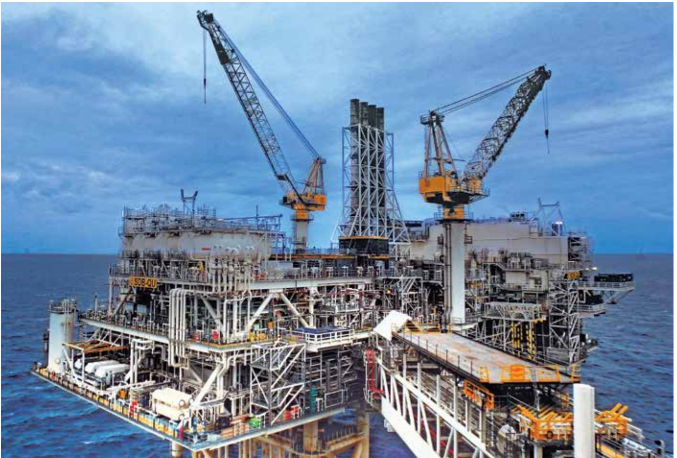
Offshore crane, Azerbaijan, Shah Deniz II
