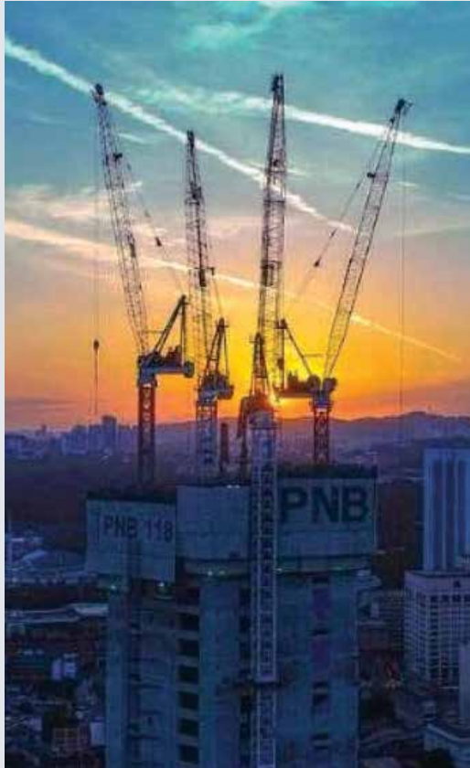
Tower CRANE, KL118, Malaysia
