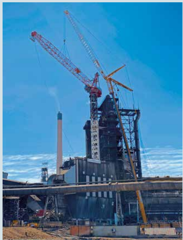
Tower Crane, Mount Isa Mines Ltd, Australia
