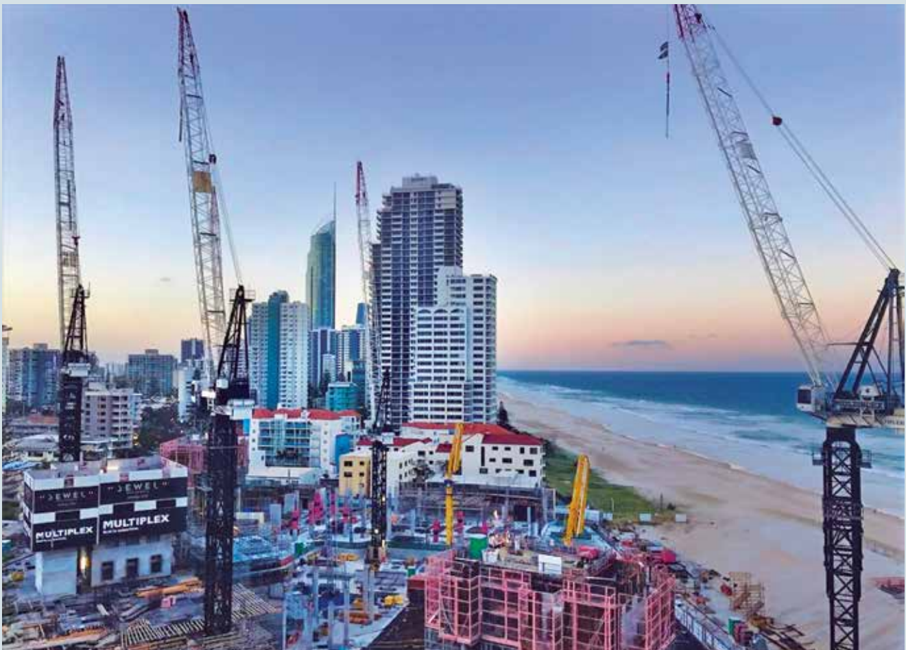
Tower Crane, Sunshine Beach Jewel Project, Australia
