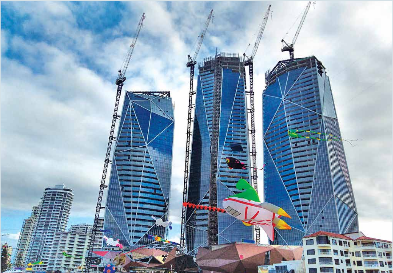
Tower Crane, Jewel Project, Australia
