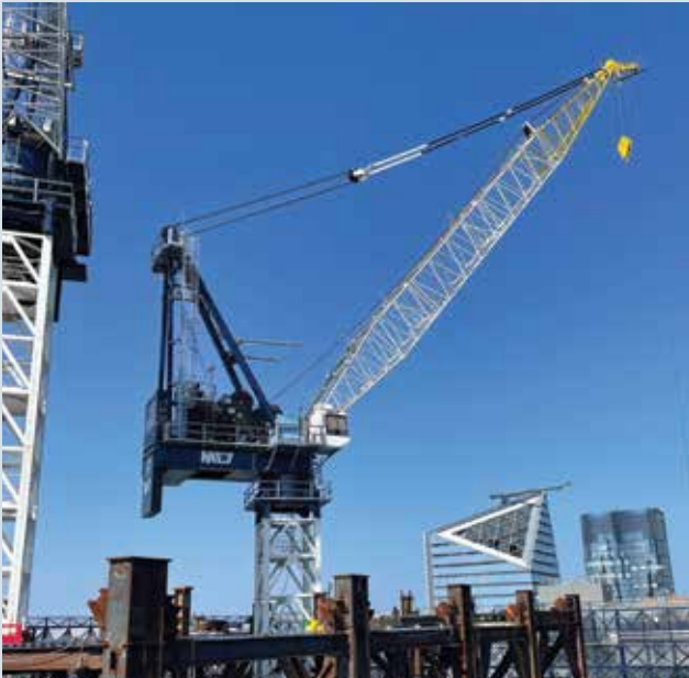
Tower Crane, New York, USA
